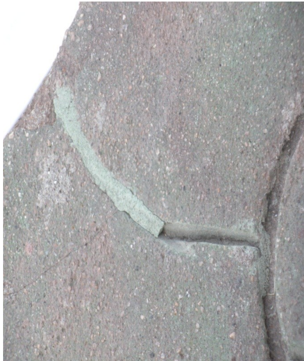
Figure 7: Loss of mortar crack fill
