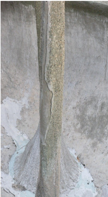
Figure 8: failed mortar repair
