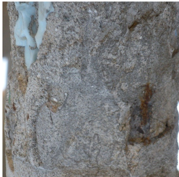
Figure 16: Cement spalling due to rust
