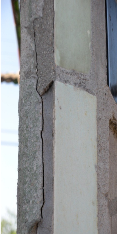
Figure 6: Loss of mortar cover over failed epoxy repair
