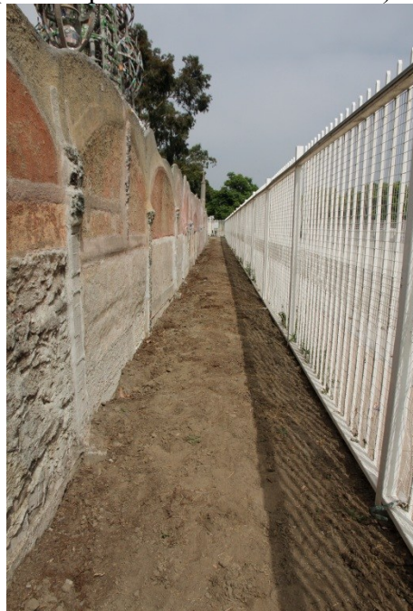
Figure 2: North side after weed removal
