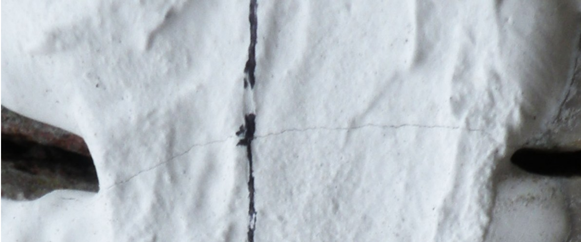
Figure 14: Crack in plaster bridge
