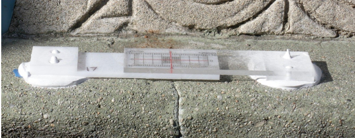
Figure 12: Telltale mounted with plaster
