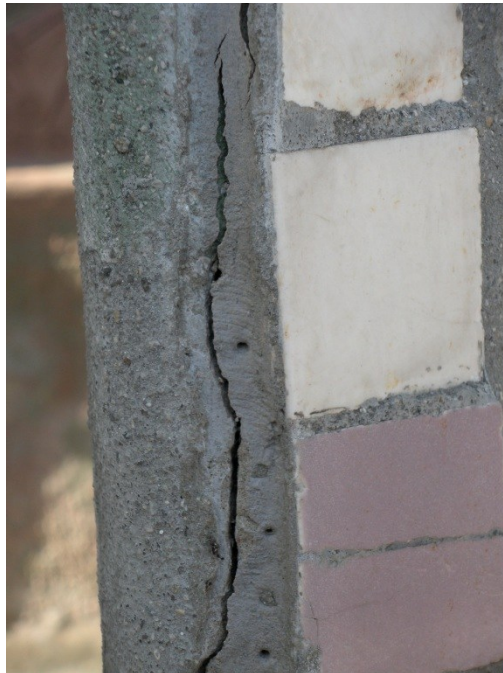
Figure 9: Cohesive failure in epoxy repair
