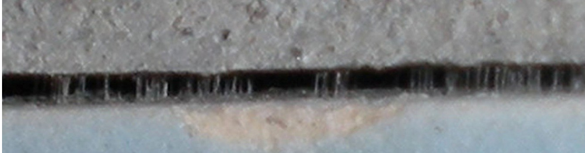
Figure 10: Cohesive failure of epoxy repair
